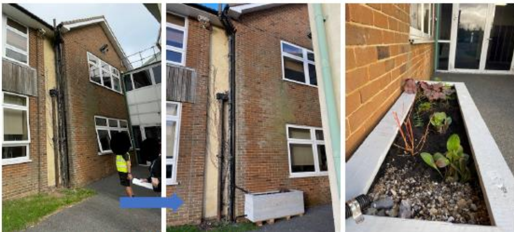
Fig.11. Images show SuDS rain -planter 6. fitted at exit route
