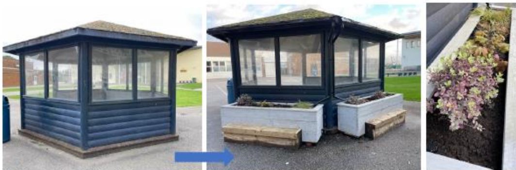
Fig.8. Images show SuDS rain -planters 1. & 2.fitted to playground shelter with seating for pupils.
