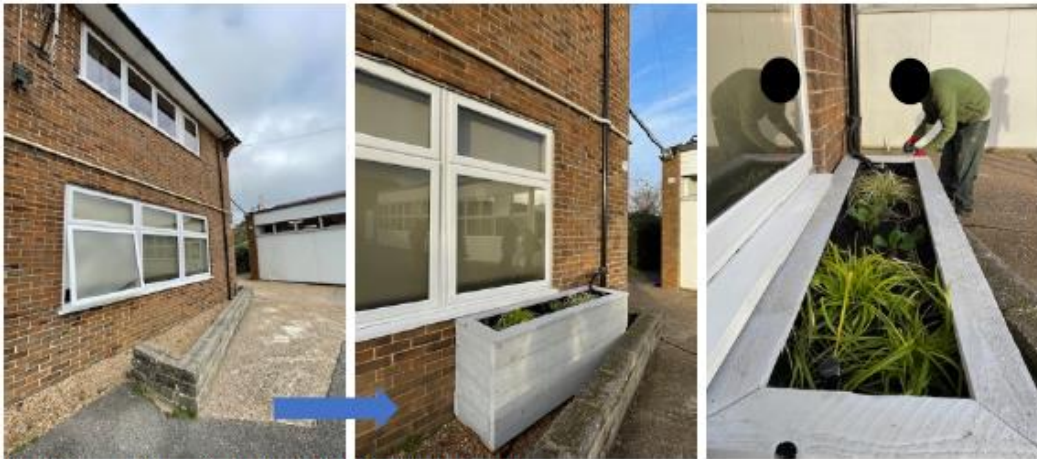
Fig. 10. Images show rain-planter 5. fitted to corner classroom
