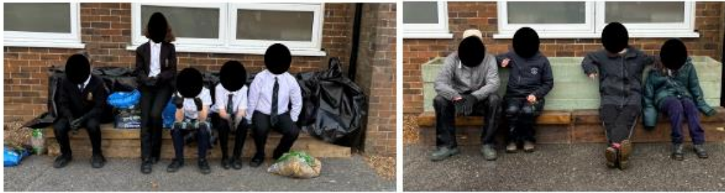
Fig. 7. Images shown pupils helping install liner and fill (a) & the new pupil seating (b)
