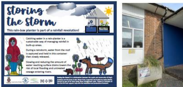
Fig. 7. Signage on the rain-planters provides on-going opportunities to engage and educate
