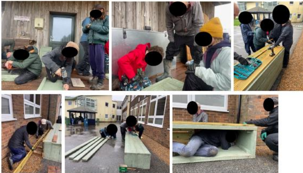
Fig. 4. Images show community construction day on 18 th November 2023
